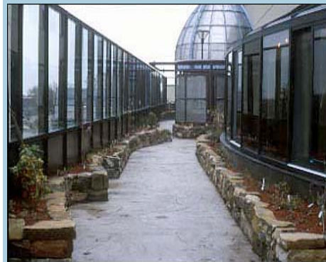
Complex Continuing Care Unit's rooftop terrace garden at Toronto East General Hospital.
